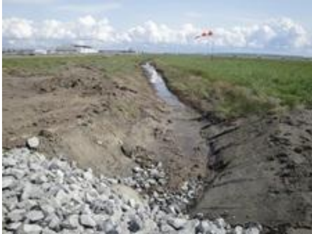
Drainage parallel to RW 07
