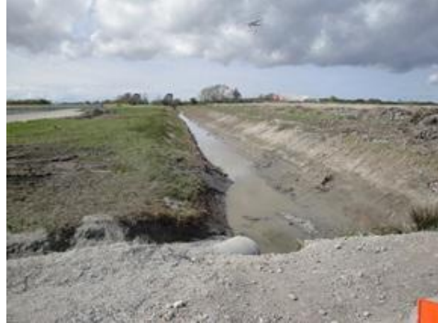
Drainage leading to 72 nd Street
